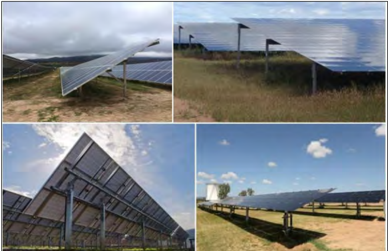
Figure 2-1: Single axis tracking mounted PV modules (ASLAT Consulting 2020: Figure 11)
