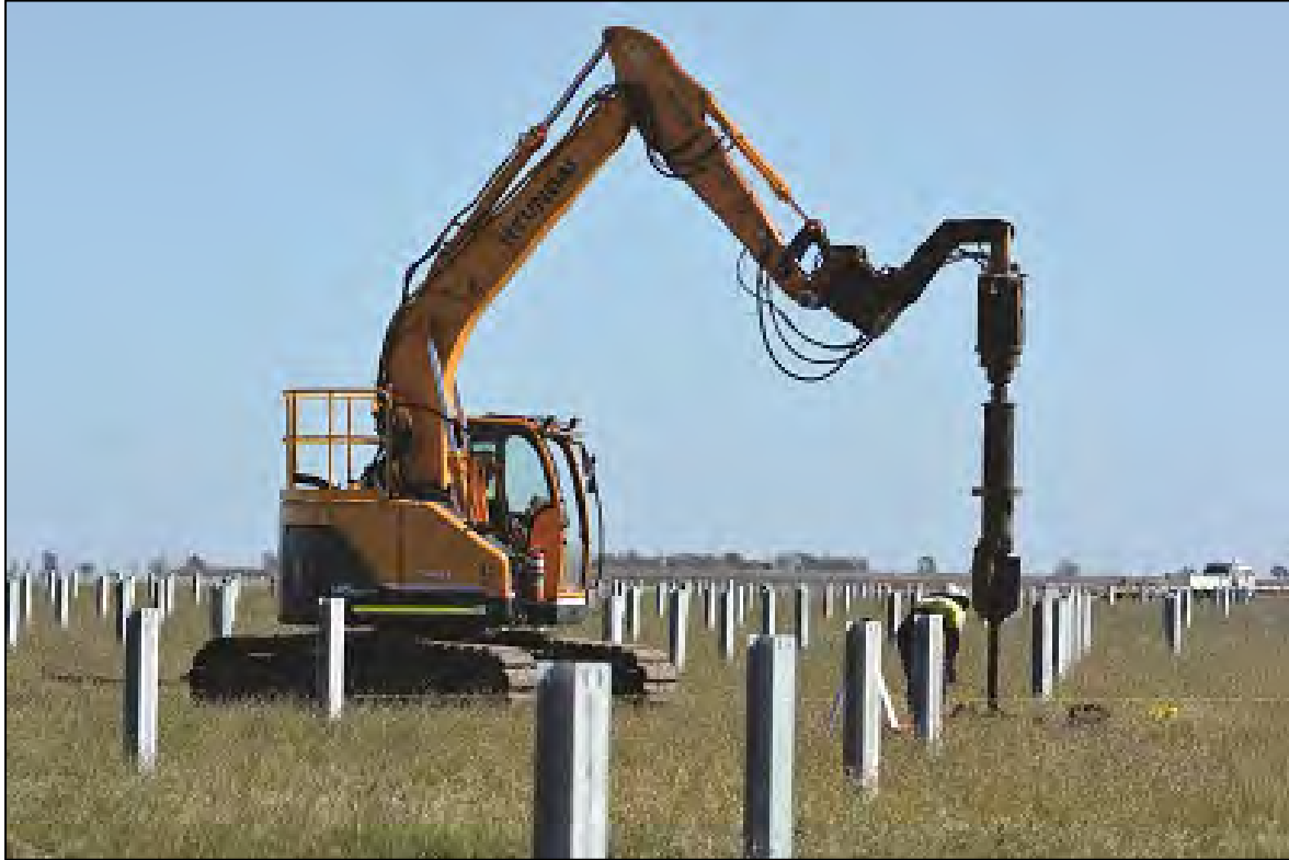
Figure 2-5: Pile driving mounting rack posts (ASLAT Consulting 2020: Figure 14)
